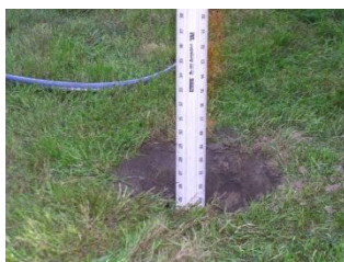
Hole for Mounting Pipe
