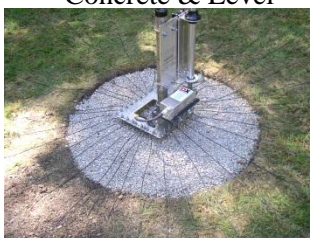
Radial Wires Installed Antenna Installed
