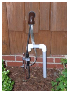
Shack end - Ground Rod and PolyPhaser protection
